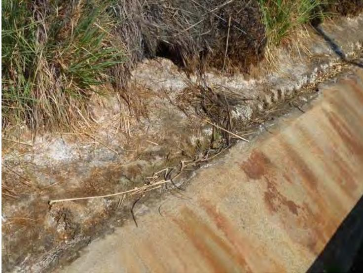
Figure 6. The slope above West Coast Highway also shows evidence of wetland conditions. This photo shows moist soils, a conspicuous salt crust, and apparent oxidation stains on the side of the concrete ditch, all indications that the groundwater seepage above Superior Avenue, shown in Figures 4 and 5, also occurs on the slope above West Coast Highway.
